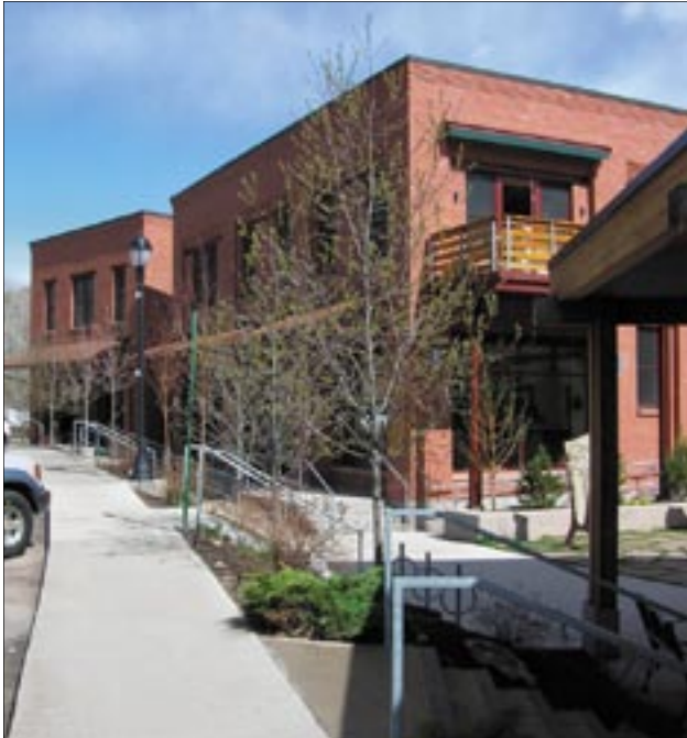
Dividing a larger building into "modules" reduces the perceived scale of the development and contributes to a human scale.
