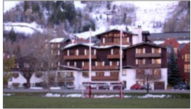
Large buildings should be designed with a base, middle and cap to reduce the perceived scale of the building.
