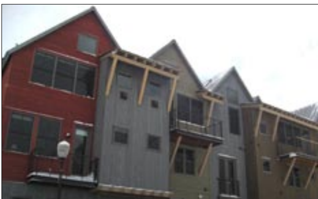
Articulating a building façade with a change in setbacks and materials helps to reduce perceived scale and convey traditional lot patterns.
