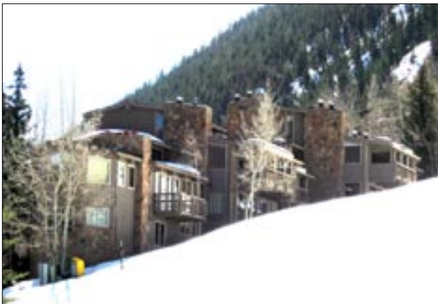
A building should be designed to reflect the change in the elevation of the site through stepped and articulated sections of the street façades.
