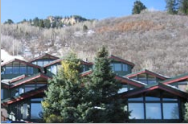
Variation in roof profile should be reflected in both the width and the depth of the roofscape of the building(s).
