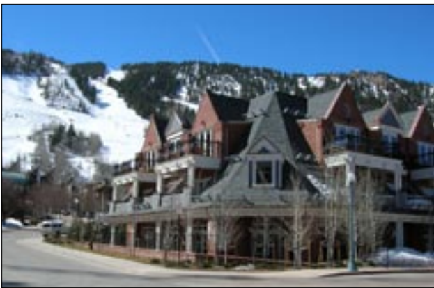
Orient a primary entrance to face the street or an area of open space adjacent to the street.
