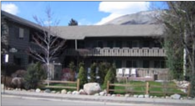
Maintain a high degree of landscaping on a lodge site.
