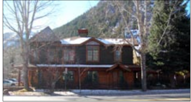
Front setbacks and mature landscaping should be maintained where a lodge is introduced into a residential context.
