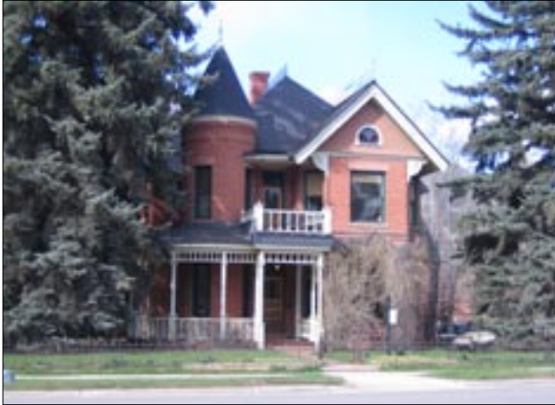
Landscaping and paving should enhance the street scene, integrate the development with its setting and reflect the quality of the architectural materials.
