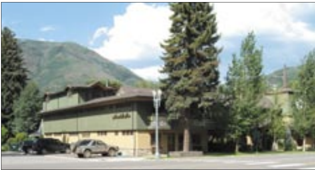
Design a building to include variation in form and profile to achieve a sense of human scale.
