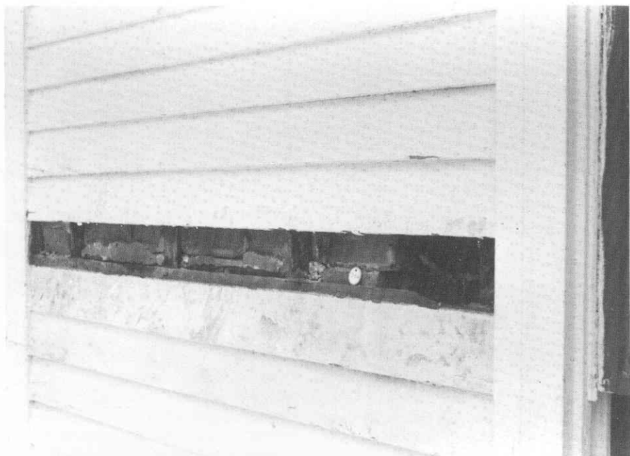
Figure 2. In assessing the safety of using thermal heat to remove paint from the siding, an investigation was performed to determine wall construction and condition. In this portion of the structure, there was no sheathing backing the siding but brick nogging extended from the foundation to the soffit. Photo: Alan O'Bright
