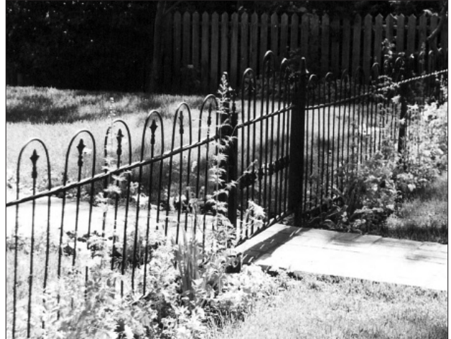
Original fences, such as this one, should be preserved.
