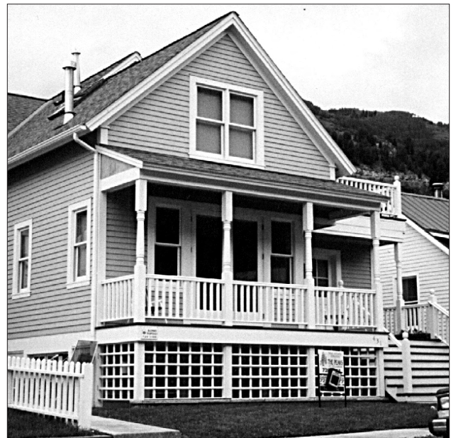
Locate the structure approximately at its historic elevation above grade. Lifting it too far up from ground level, such as in this example, is inappropriate.
