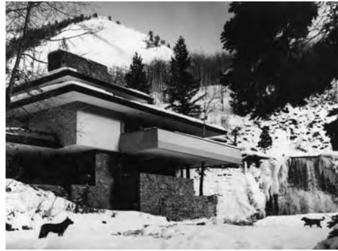
Waterfall House, on Castle Creek Road, Pitkin County, 1960
