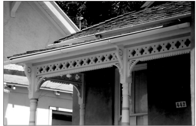
Wood detailing on porches, such as this jigsaw ornamentation, should be preserved.
