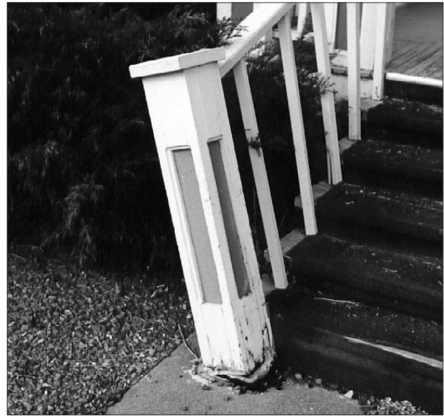
Because of constant exposure to sun and rain and the fact that a porch is open to the elements, it decays faster than other portions of a house.
