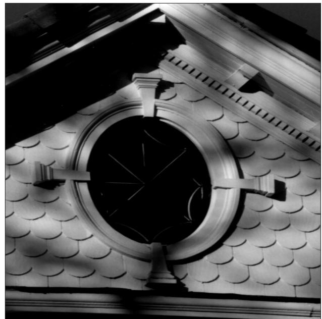
Ornamental windows such as those above are character-defining features that often indicate the architectural style of a house.
