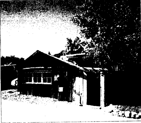
A historic outbuilding adapted for use as an architect's office.
